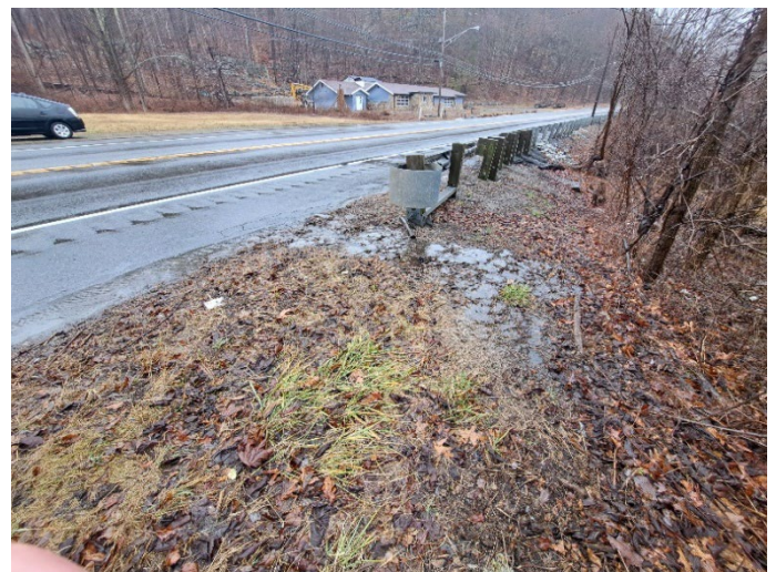
Photo 8-65: Storm runoff rills in front of guardrail toward wetland complex (Recommendation 33B)
