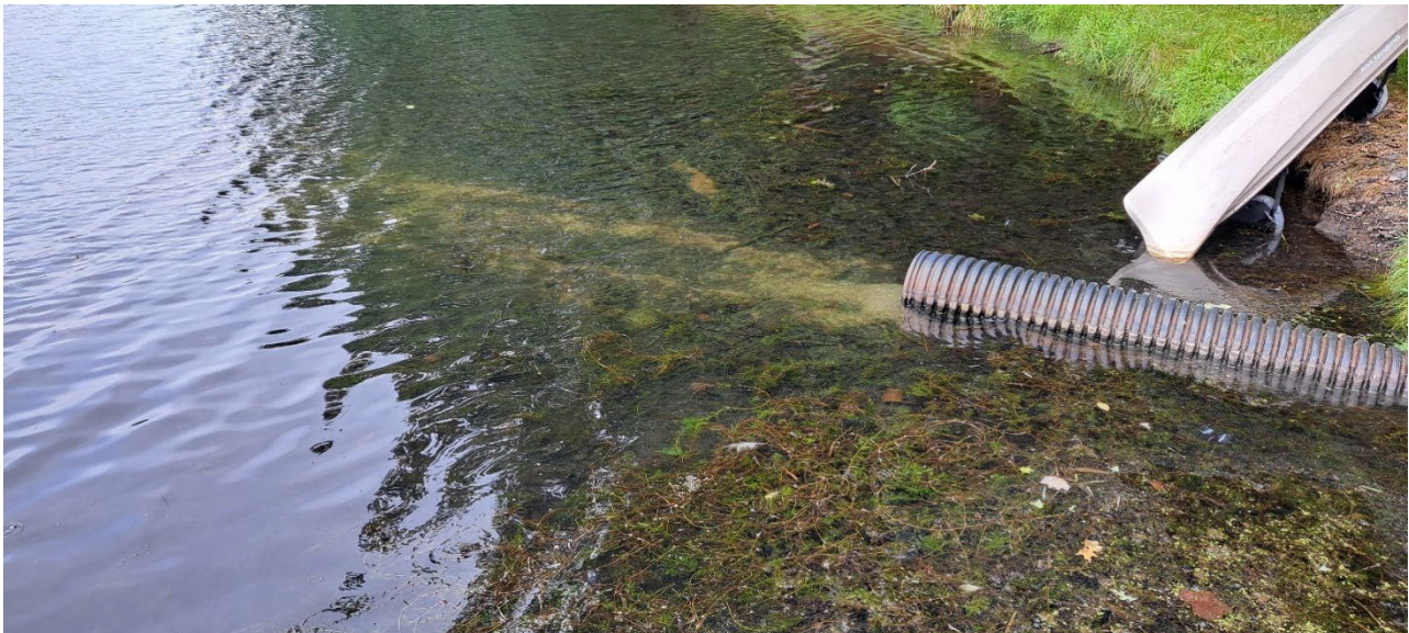
Photo 8-48: Sediment can be seen at the end of the stormwater pipe discharging from the adjacent parking lot. The pipe was also laden with gravel and sediment
