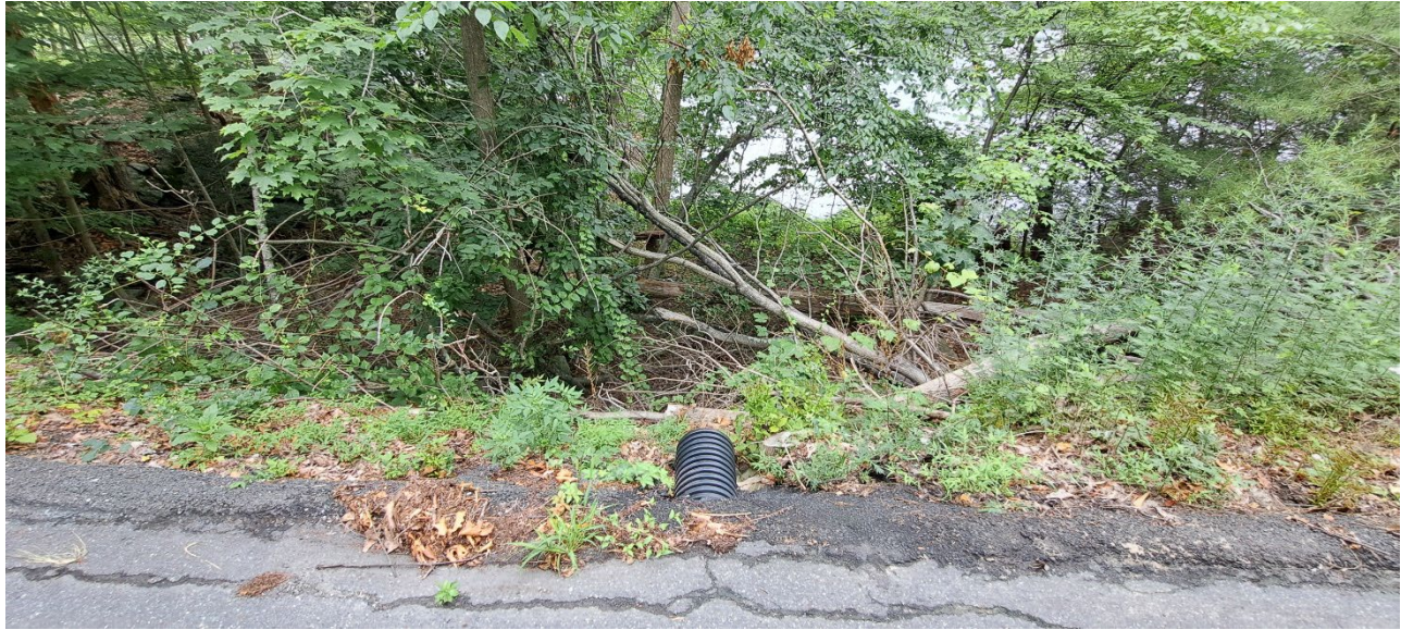
Photo 8-52: Discharge pipe causing a moderate amount of erosion below the pipe
