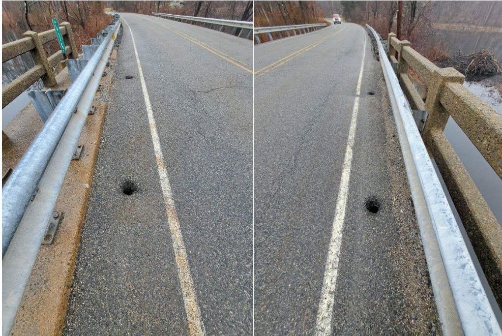
Photo 8-56: Holes to drain road runoff directly into Wolf Lake (Recommendation 30B)
