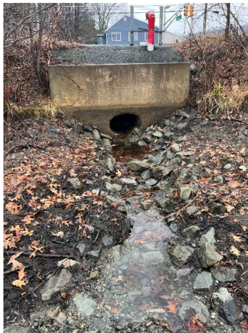
Photo 8-3: The drainage from the swale across Route 206 (Recommendation 2B)
