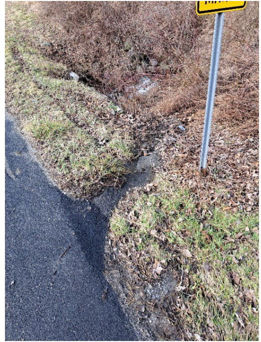
Photo 8-29: Rill draining into an un-named tributary eroding along Sparta Rd (Recommendation 17A)
