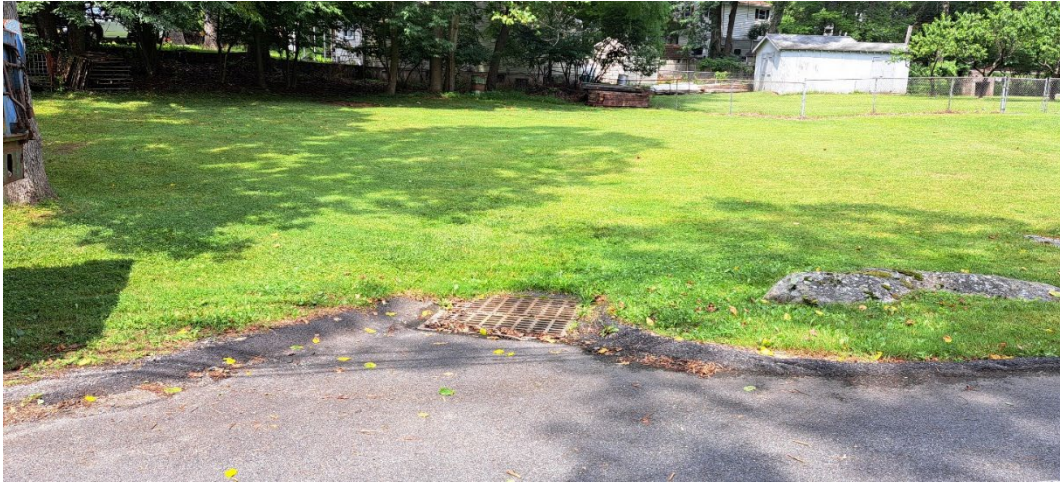
Photo 8-9: Catch Basin along N Shore Rd that is suitable for a roadside rain garden
