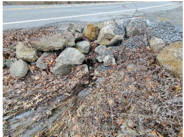
Photo 8-37: The culvert is being partially blocked by the riprap and is becoming clogged with driveway material and plant matter (Recommendation 19A)
