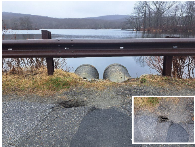
Photo 8-70: View of the overflow culverts looking toward Jefferson Lake. The inset is an overhead view of the hole in the road deck that drains into the culvert on the left (Recommendation 35C)
