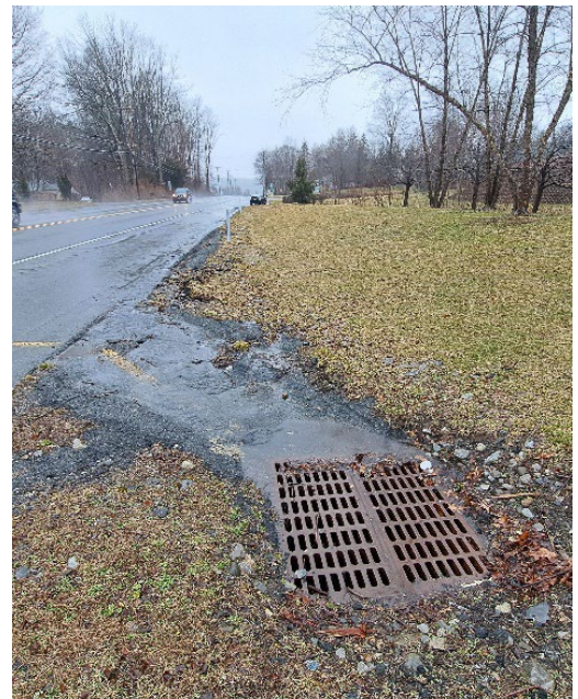
Photo 8-67: Stormwater Runoff along Rt 206 North in front of Metro Self Storage (Recommendation 34A)
