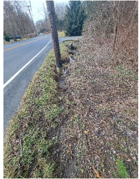
Photo 8-33: Active erosion around utility pole from stormwater runoff (Recommendation 18B)
