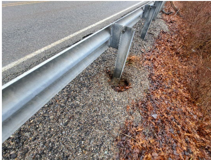
Photo 8-55: Scour hole is being formed along the guardrail support from stormwater runoff (Recommendation 30A)
