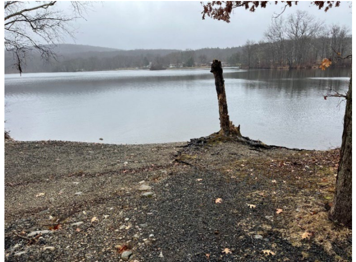
Photo 72: Existing snag and erosion along the Jefferson Lake boat launch (Recommendation 36A)
