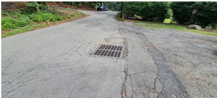
Photo 8-10: Standard catch basin along Hightoga Trail
