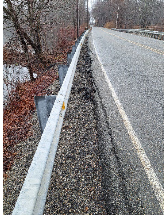
Photo 8-54: Shows edge of road degrading from surface runoff and gravel washout (Recommendation 30A)
