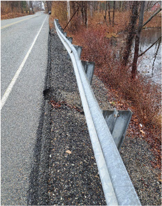
Photo 8-53: Erosion forming along the Roseville road base (Recommendation 30A)
