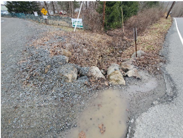
Photo 8-36: View of driveway material being plowed into the drainage swale (Recommendation 19A)
