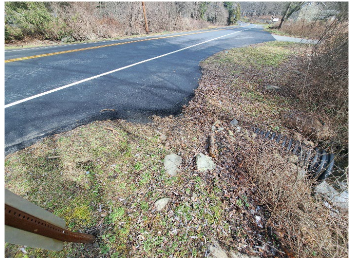
Photo 8-35: Misaligned channel and bank erosion along culvert headwall (Recommendation 18B)
