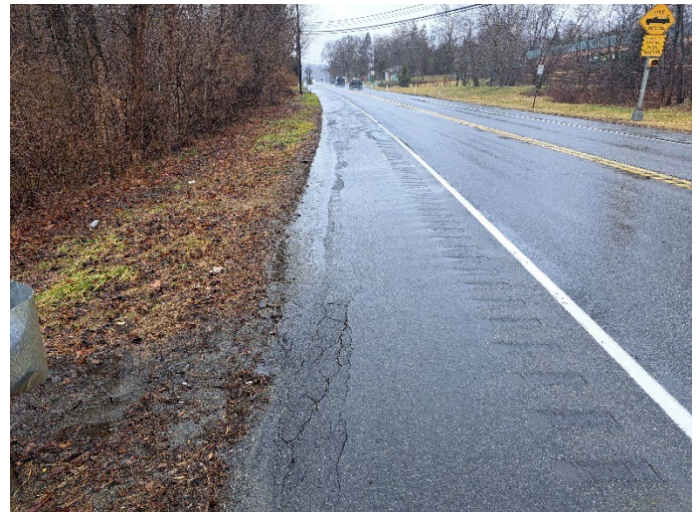
Photo 8-63: Storm run-off runs along the shoulder of Rt. 206 (Recommendation 33A)
