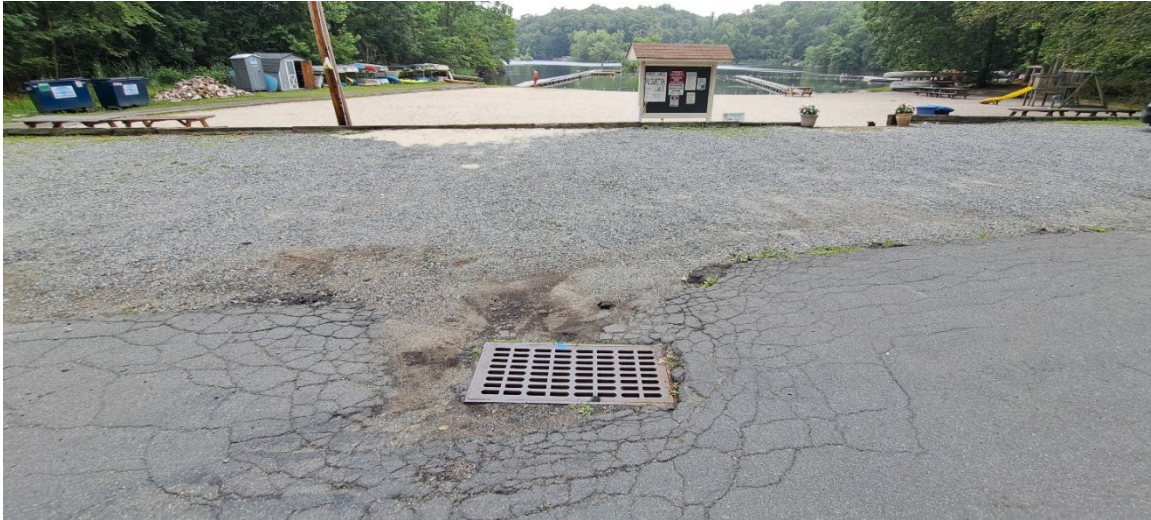
Photo 8-51: Catch Basin in front of the southern beach with signs of erosion and sediment near the inlet grate
