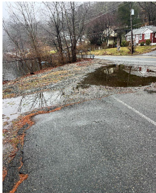
Photo 8-189: The south end of the parking lot with excess road gravel and pooled water (Recommendation 12B)
