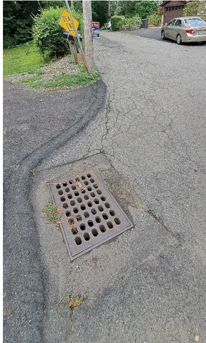
Photo 8-8: Standard Catch Basin along Division Ln
