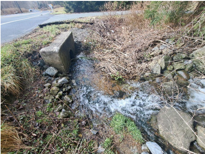
Photo 8-34: Downstream section of culvert showing exposed HDPE pipe and potential for erosion along edge of the road (Recommendation 18B)
