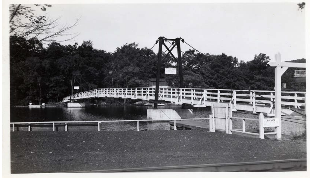
1937 Morris Canal Abandonment Cranberry Lake Suspension Foot Bridge
