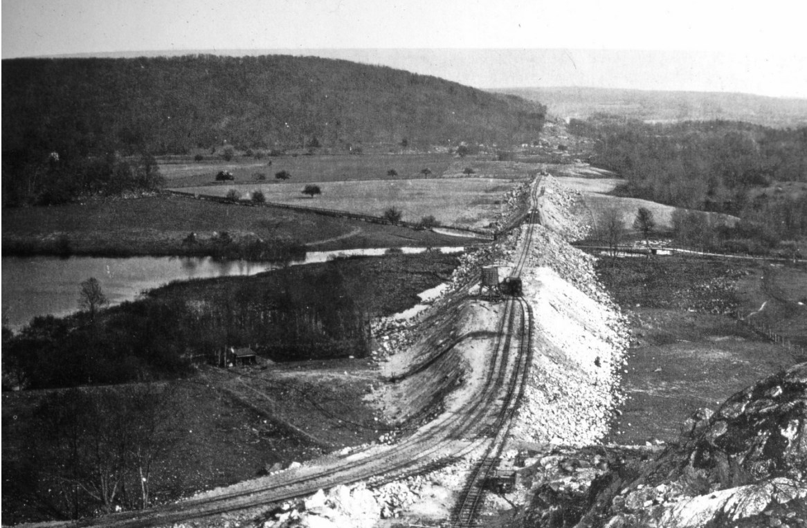
1910 Lackawanna Cut-off Warton Fill over Roseville Road
