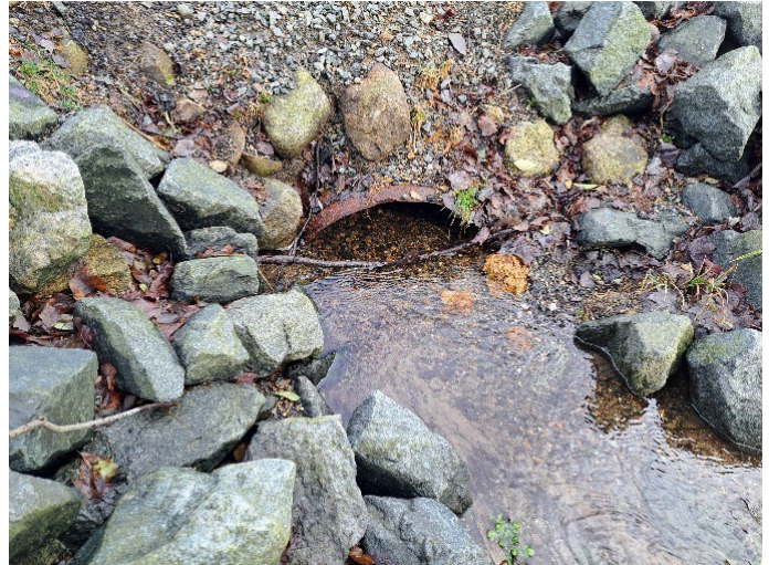
Photo 8-19: Downstream side of culvert (Recommendation 24A)
