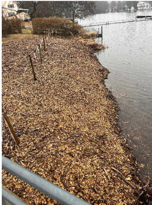
Photo 8-32: The mulched shoreline of the recreational area near the Lackawanna dam (Recommendation 13A)
