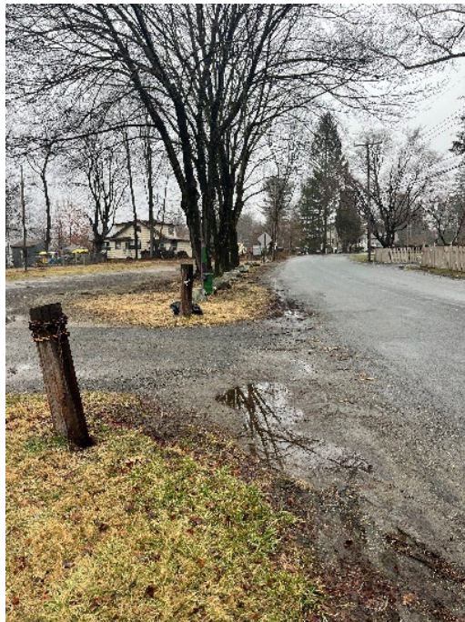
Photo 8-36: The area where the parking lot meets Lake Dr (Recommendation 15C)
