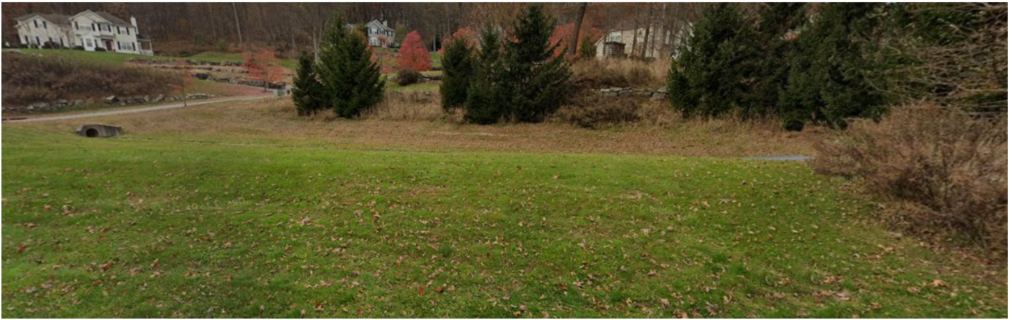
Photo 8-16: Northern retention basin at intersection of Ascot Ln and Sparta Rd (Recommendation 7A)
