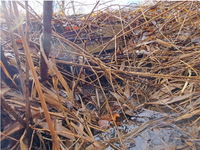
Photo 8-18: Upstream side of culvert (Recommendation 24A)
