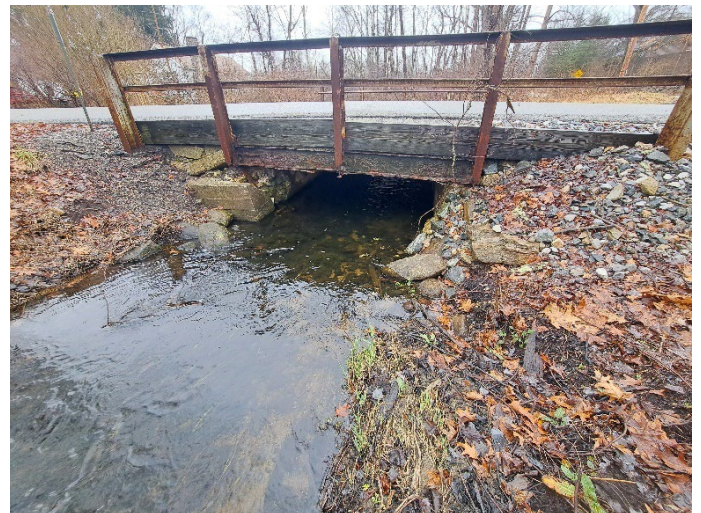
Photo 8-43: S Shore Rd bridge crossing [Site Outlet] (Recommendation 18C)
