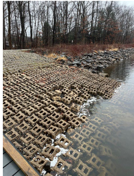
Photo 8-7: Cranberry Lake boat ramp (Recommendation 4A)
