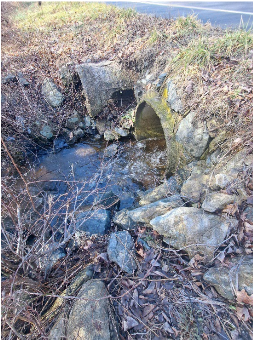
Photo 8-13: Upstream view of culverts that cross under Sparta Rd (Recommendation 6A)
