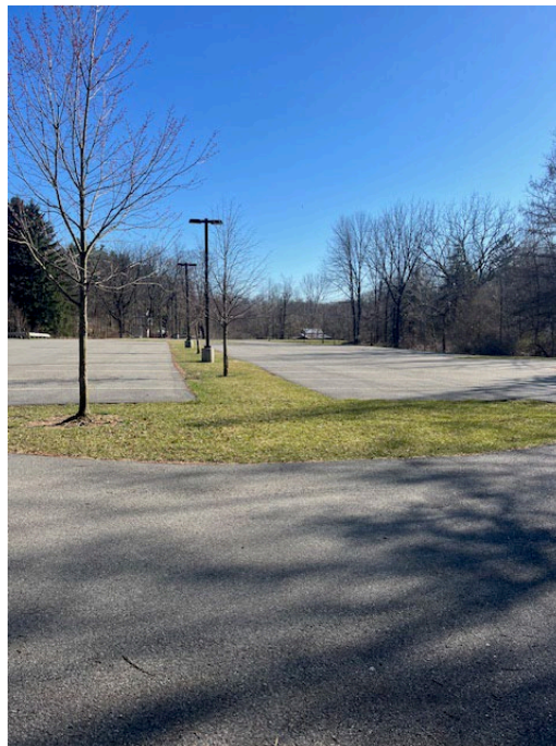
Photo 8-1: The western parking lot at Tamarack Park (Recommendation 1A)
