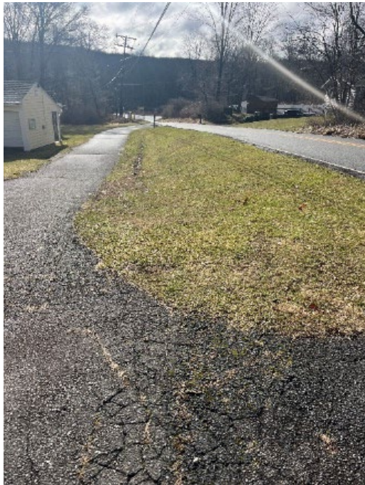
Photo 8-9: The grass area between Seneca Rd and the paved roadway to the parking lot (Recommendation 5B)
