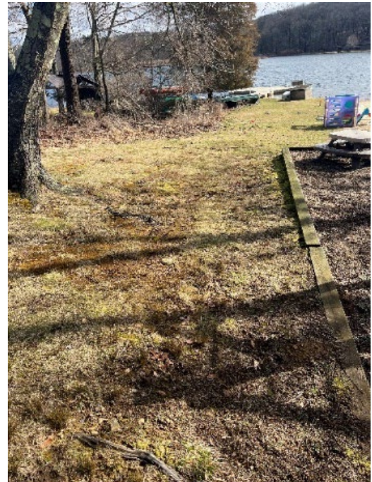
Photo 8-10: Erosion along the northwest side of the playground located in the beach area (Recommendation 5C)
