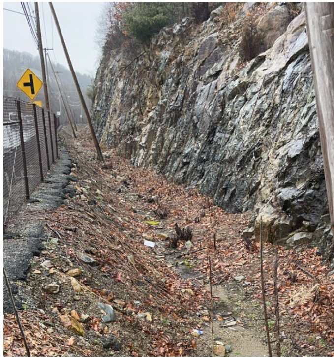
Photo 8-2: Swale that runs alongside Route 206 N (Recommendation 2A)
