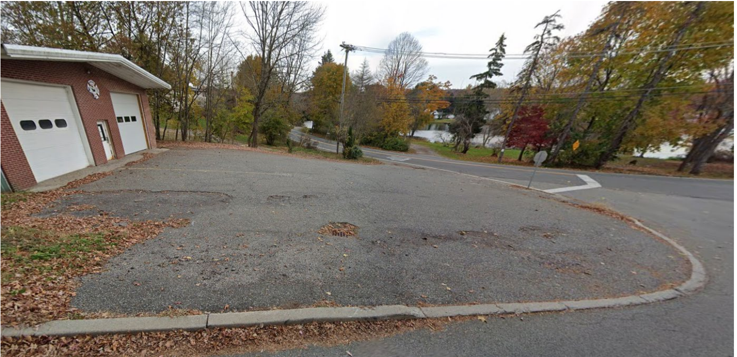
Figure 8-23: Byram Fire Department Parking lot as seen from Roseville Rd (Recommendation 9A)
