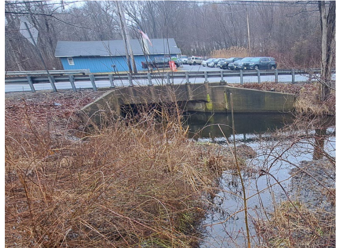
Photo 8-41: 206 crossing of Ghost Pony Brook [Site Inlet] (Recommendation 18A)
