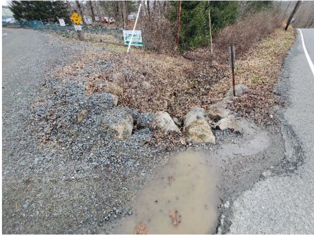
Photo 8-21: View of driveway material being plowed into the drainage swale (Recommendation 8A)
