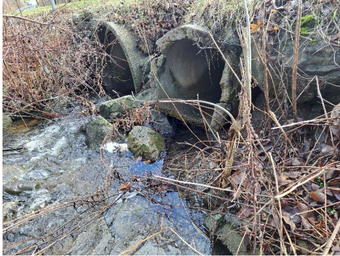
Photo 8-12: Upstream view of culverts that cross under Sparta Rd (Recommendation 6A)
