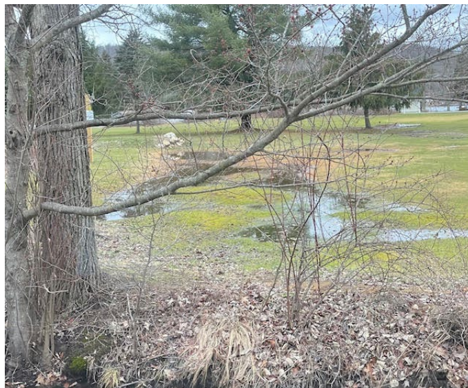
Photo 8-37: Standing water behind the 1st green on the Lackawanna golf course along Reis Ave (Recommendation 16A)
